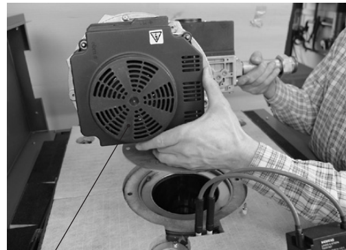
Fan and gas mixing device
